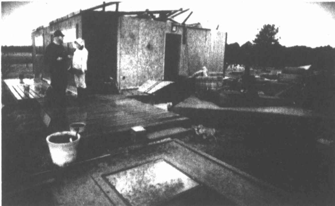
Bob and Betty Watson stand on porch of damaged home.
