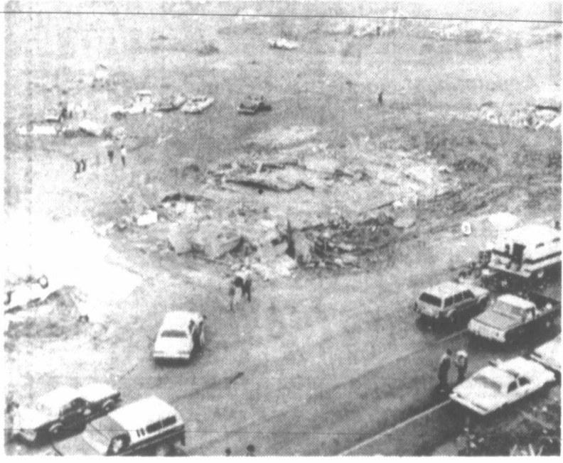
Only twisted rubble remains.
