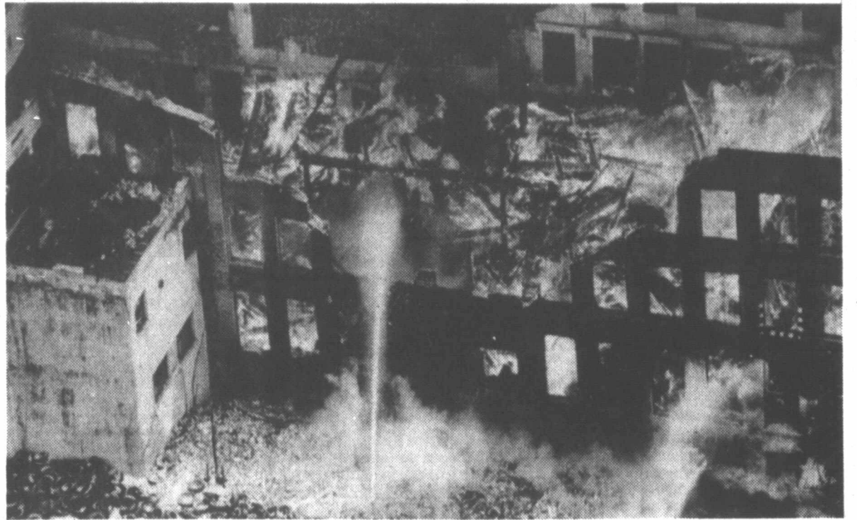
Detroit warehouse destroyed by fire.
