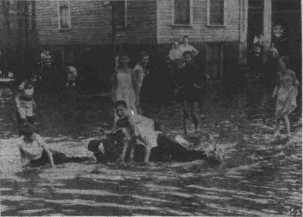
Flooded Street Their Swimming Pool
