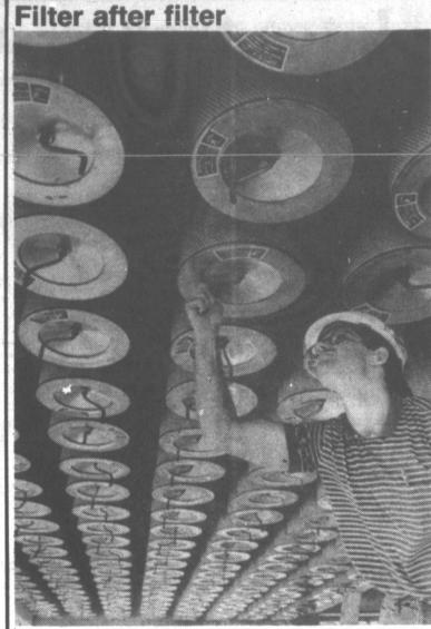
A maintenance man checks air filters at the PPG Industries chemical plant in Lake Charles, La. Air pulled through the filters combusts with natural gas to power turbines that create power for the manufacture of chlorine and caustic soda.
