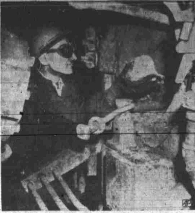
Steel Furnace Plugged
