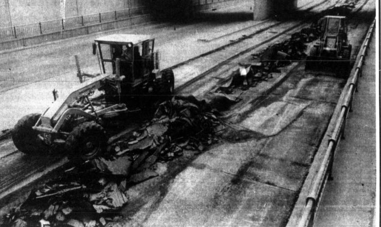
Road graders with Lewis Construction Co. strip asphalt on Hobart Street at the Santa Fe railroad tracks. The Texas Department of Highways and Public Transportation is resurfacing Hobart, the route of Texas Highway 70, replacing traffic lights and upgrading intersections. Department officials estimate that the project will cost \$387,754 and anticipate completion by the early part of October. (Staff Photo by Terry Ford)
