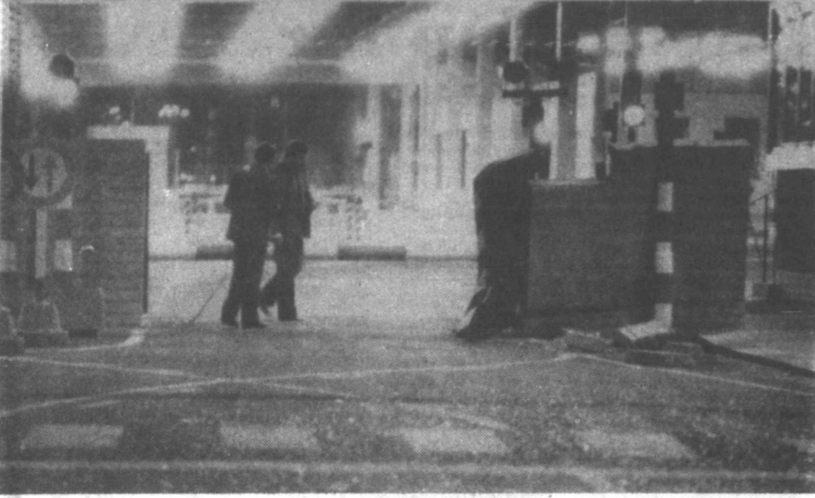
ESCAPE THROUGH THE WALL — East German officials during the securing of evidence at Checkpoint Charlie, after three people escaped across the Berlin Wall early Friday with a truck through a barrier. At right is destroyed piece of the wall and gate, in the foreground splinters of glass of the truck windshield. (AP Laserphoto)
