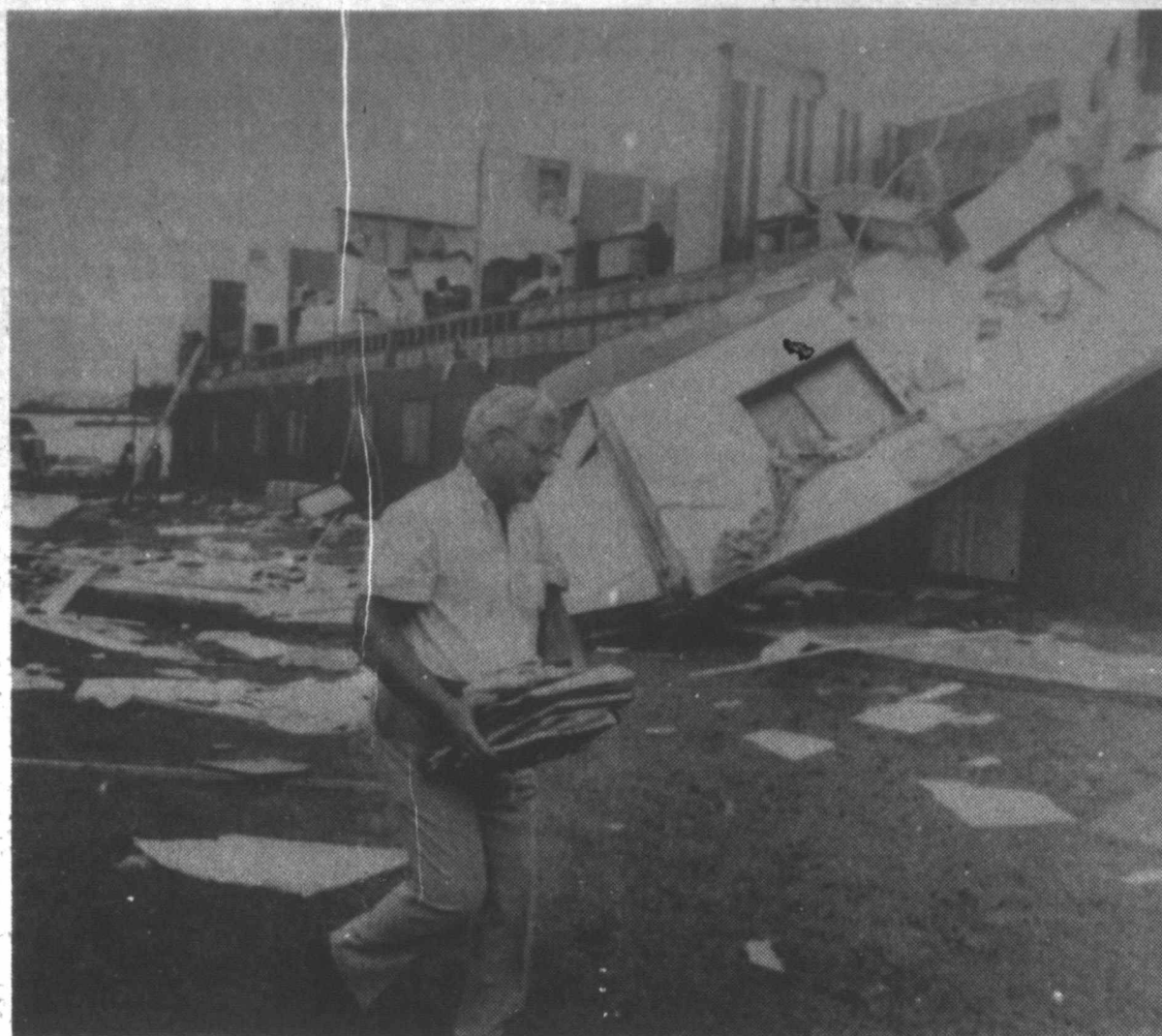
TORNADO DAMAGE — George Mills, owner of Mills Insulation in West Des Moines, Iowa, carries company records away from his tornado damaged offices early this
