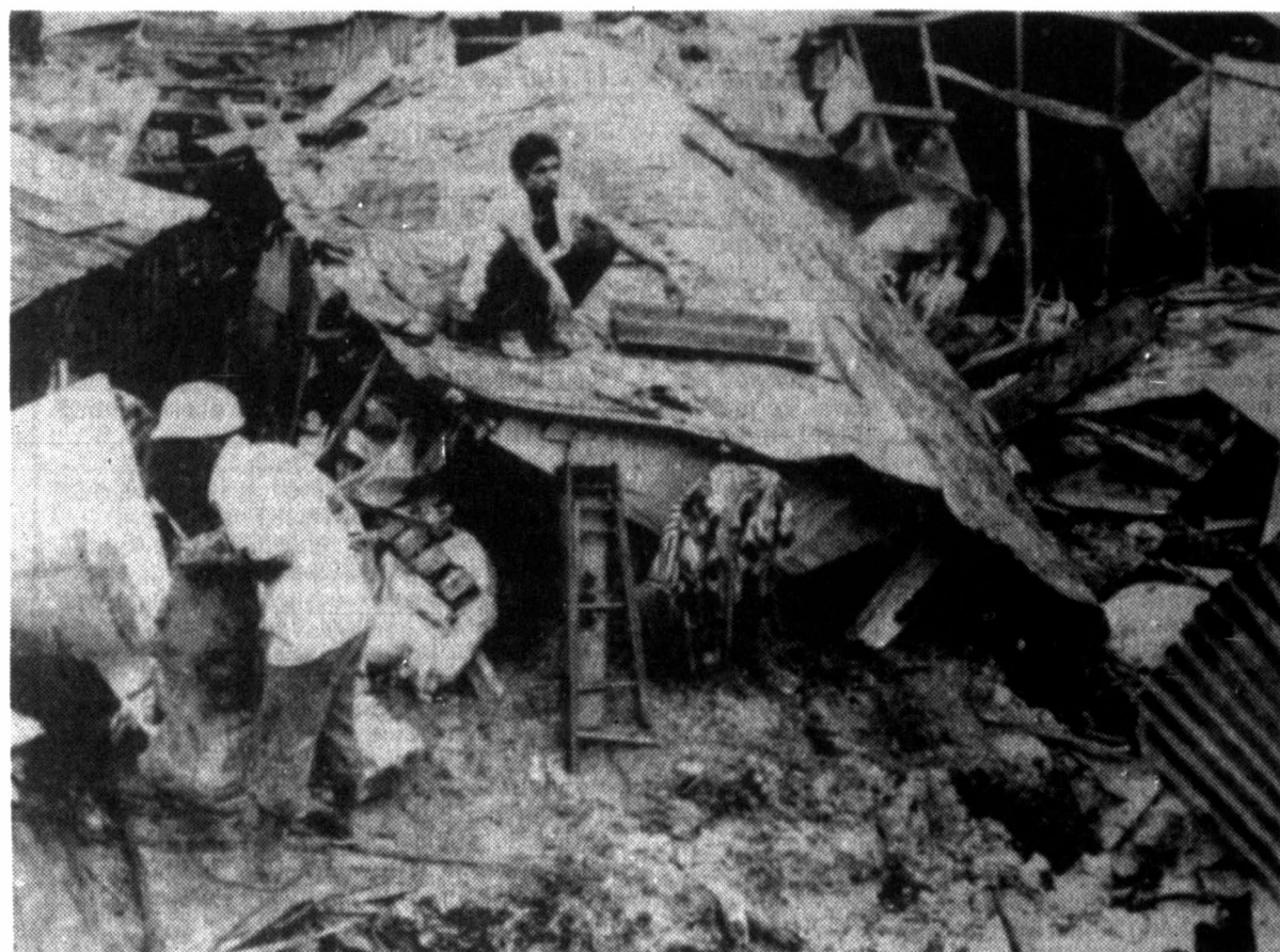
RAIN DAMAGE — A man tries to reach his belongings while another man surveys damage from the roof of a house which was destroyed by rains in the Dominican Republic during the past five days. Fifteen people have died in the Dominican Republic and Haiti as a result of the flooding, according to police. (AP Laserphoto)
