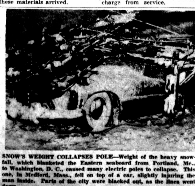
SNOW'S WEIGHT COLLAPSES POLE—Weight of the heavy snowfall, which blanketed the Eastern seaboard from Portland, Me., to Washington, D. C., caused many electric poles to collapse. The one in Medford, Mass., fell on top of a car, slightly injuring the man inside. Parts of the city were blacked out, as the lines went down.
