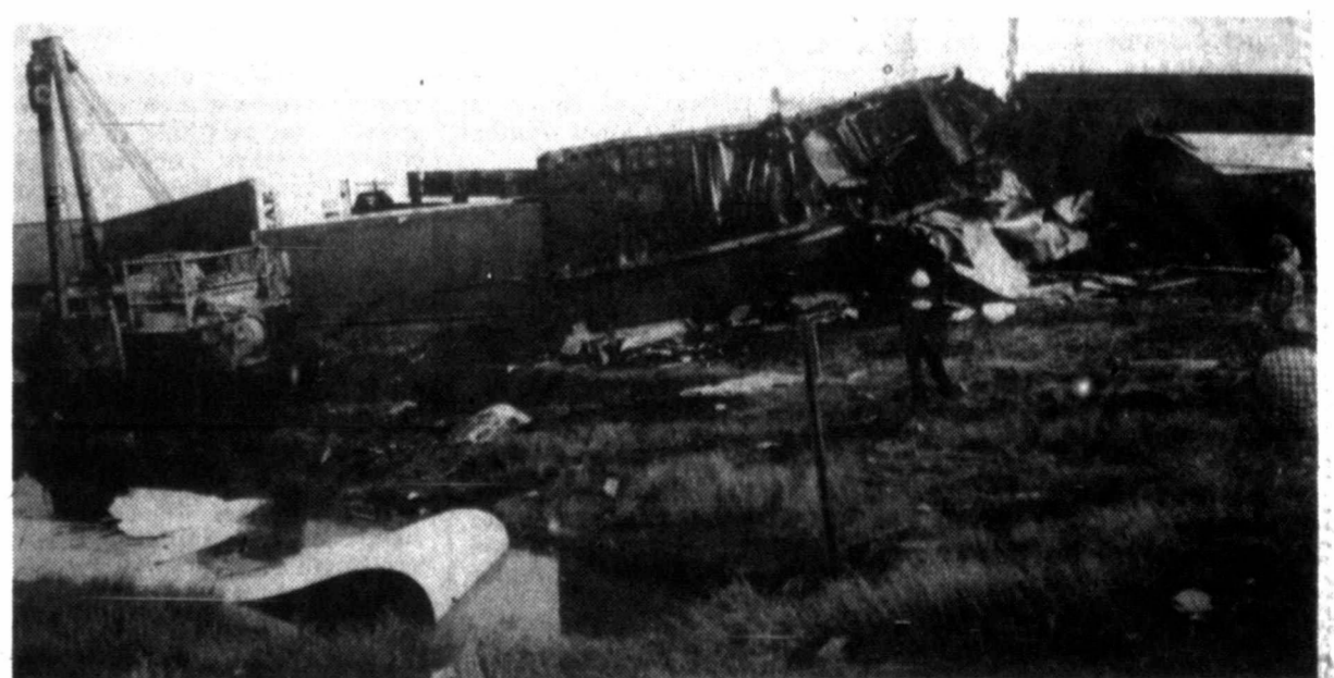
DIRECTING TRAFFIC — A foreman from Hulcher Emergency Service of Amarillo points to the driver of a bulldozer working to untangle one of the approximately 60 Santa Fe Railway cars that derailed west of
