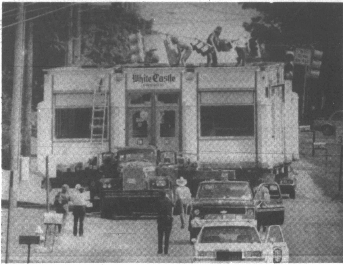
RESTAURANT DRIVE-AWAY — Traffic lights had to be held up, as did motorists, for a time Sunday while workers moved this 35-year-old restaurant building from a busy in-
