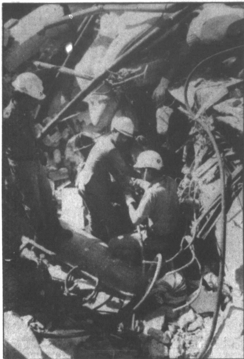
RESCUE EFFORTS CONTINUE —Rescuers work Sunday in the rubble that was the New World Hotel in Singapore. The hotel collapsed "like a deck of cards" Saturday, killing at least six persons. As many as 100 could still be trapped in the debris. (AP Laserphoto)
