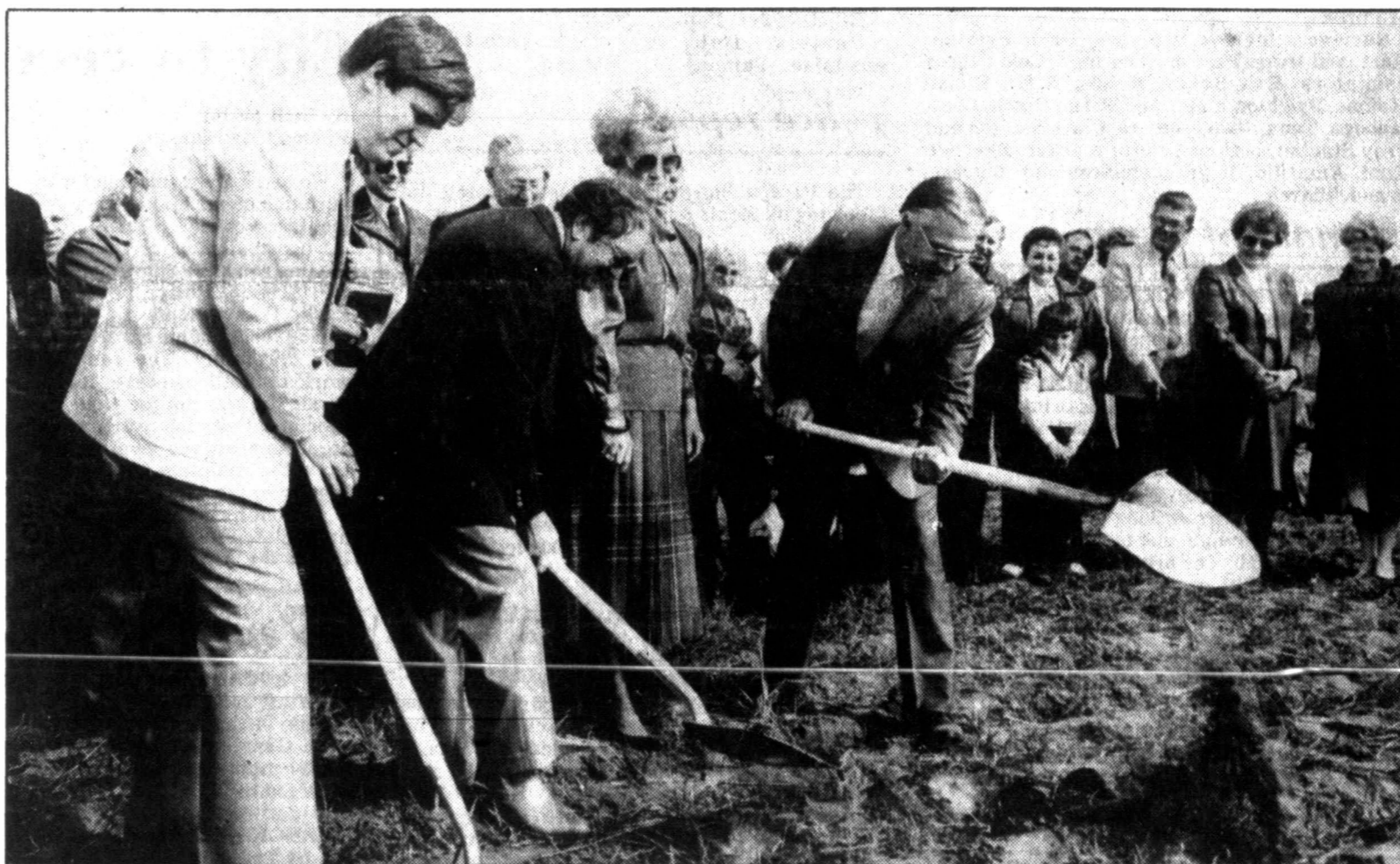
NEW CHURCH CENTER - The congregation of Lamar Full Gospel Assembly gathered Sunday afternoon at Harvester and Lynn for groundbreaking ceremonies for construction of their new $1.2 million church and family life center. Turning over the first shovelful of dirt are, from left, City
