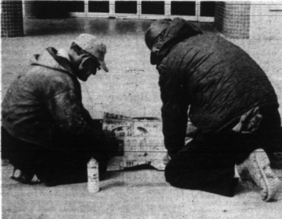
MAKING IT CLEAR —Employees of the Pampa Street Department have been repainting fire lane areas on curbs within the city to make it easier for residents to see. Painting a "fire" sign on the curb in front of the Capri Theater—see from left, Leslie Edmondson, 511 N. Roberta, and G.D. Minyard, 1005 S. Faulkner. The painted areas are to be left clear in case of fire emergency use. (Photo by Doug Abbott)
