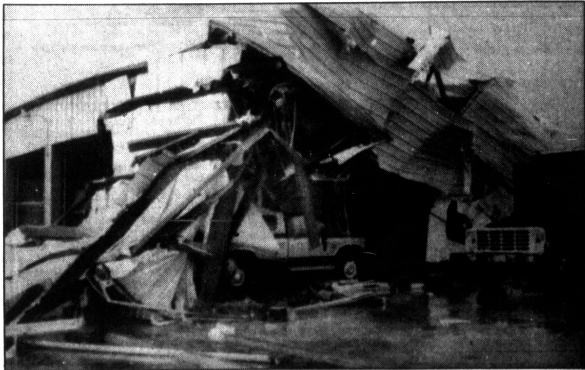
Tornado leaves Houston building in shambles
