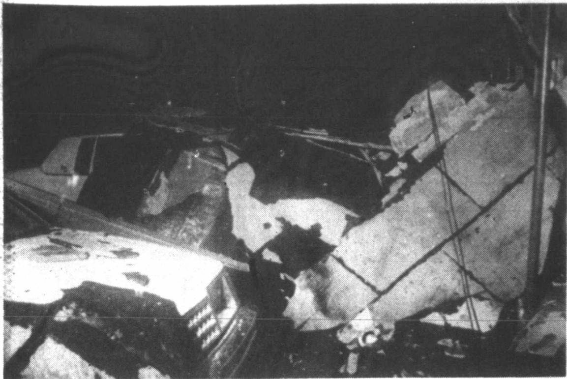
STORM DAMAGE — Parts of the roof of a motel lot Thursday near Panama City, Fla., motel cover the hoods of cars parked in the following the landfall of Hurricane Kate.
