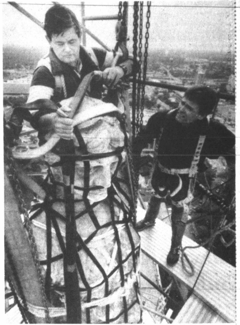
PREPARE FOR LIFTOFF — State Architect Roy Graham, right, and Pat Rice check lift lines on the Goddess of Liberty Statue atop the Texas Capitol. She is scheduled to come down by helicopter Sunday in preparation for her replacement with a replica. (AP Laserphoto)
