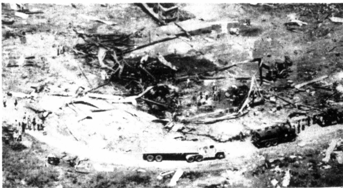
Only debris remains at plant site
