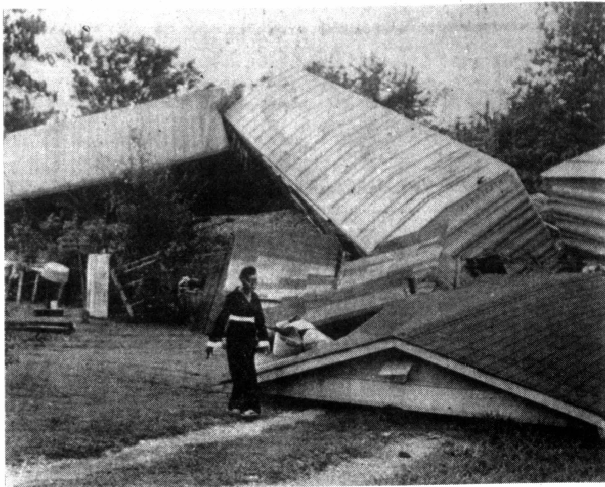
TRAIN HITS GARAGE —Ella Cole of Stevenson, Ala., surveys her destroyed garage this morning after seven cars of a Seaboard System Railroad derailed in her backyard
