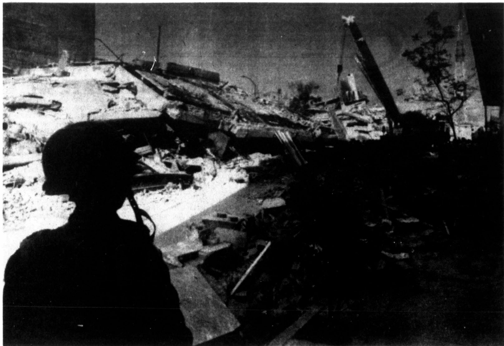
KEEPING GUARD —A Mexican soldier looks over the rubble of an apartment house in Mexico City leveled by an earthquake Thursday. A crane works at removing slabs of concrete as workers look for victims. (AP Laserphoto)
