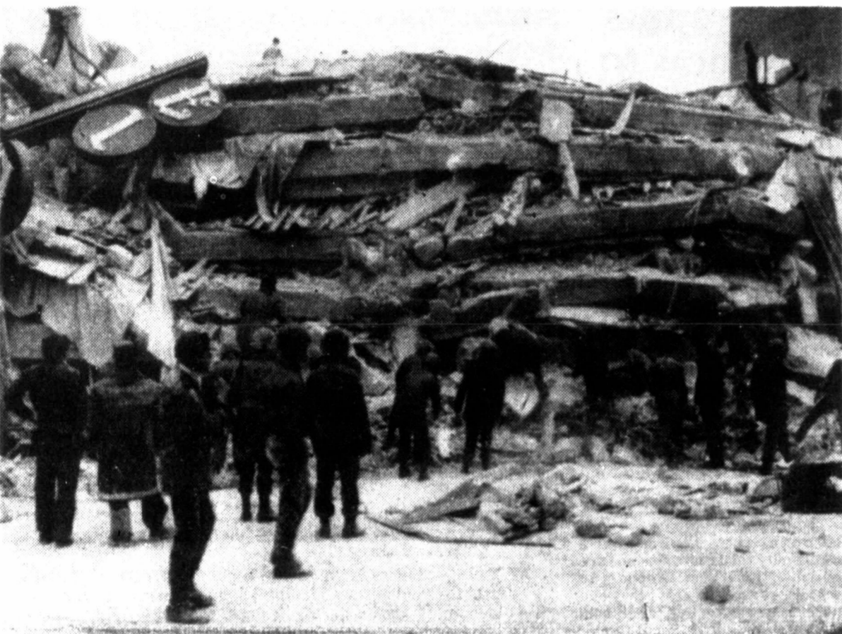
REMAINS OF HOTEL—Rescue workers search through collapsed floors of a Mexico City hotel that are piled on top of each other like a stack of pancakes after the two earthquakes that hit the area Thursday and Friday. (AP Laserphoto)
