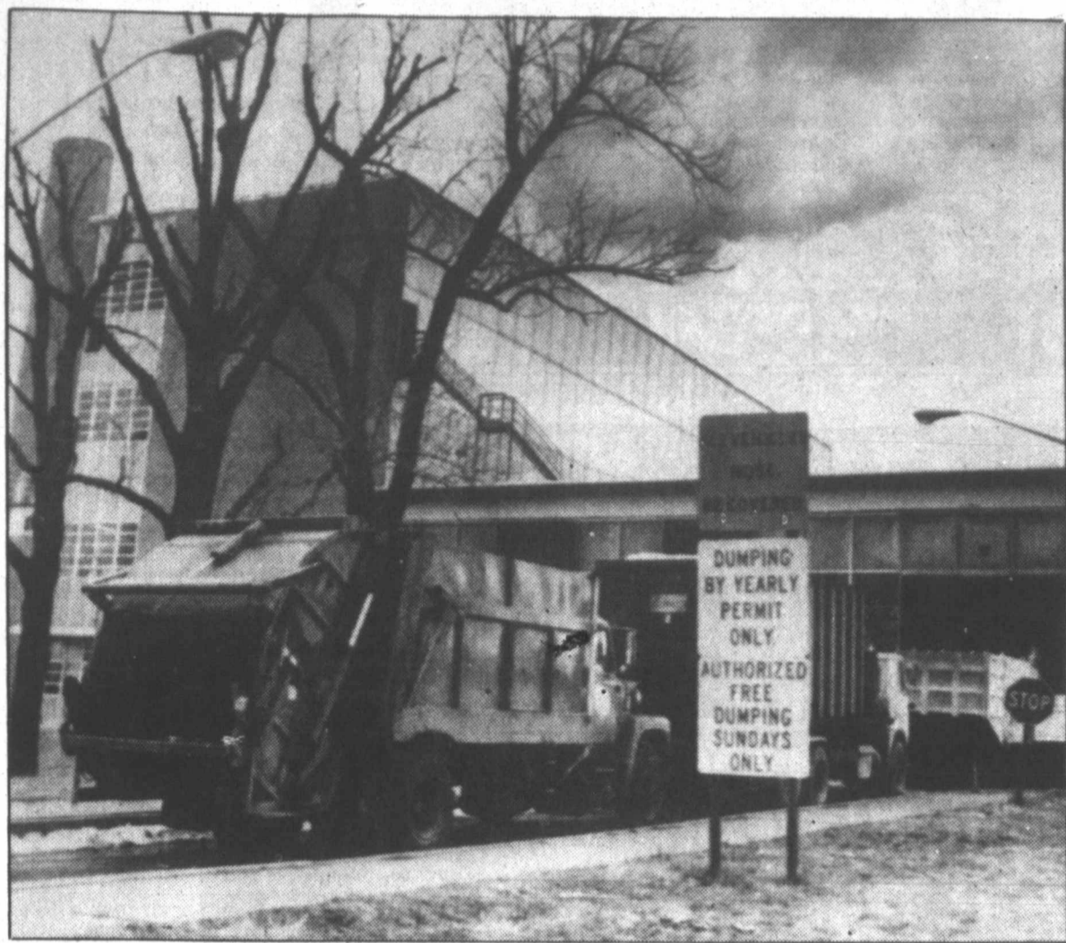
TRASH PLANT —Garbage trucks are shown in line at the Harrisburg, Pa., incinerator recently as they wait to be unloaded. Municipal officials and engineers from around the world come to
