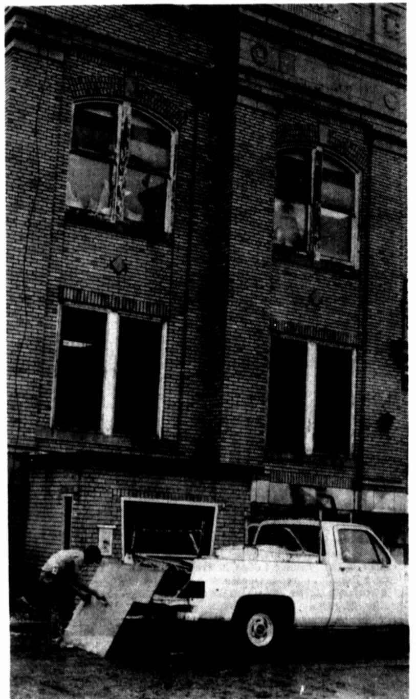
WINDOW BOARDS —A workman at city hall measures more material to temporarily replace broken windows at city hall after boarding up the two shown on the second floor. (Staff photo by Wally Simmons)
