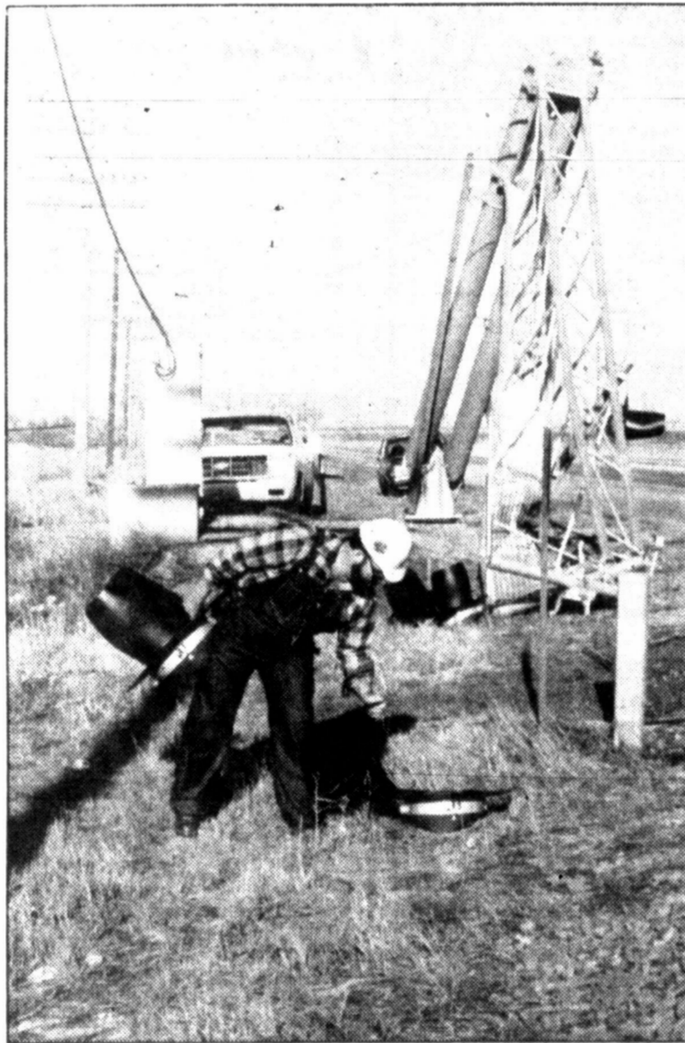
WRECKAGE CLEAN-UP — Rick Tackett, an employee with Santa Fe Railroad picks up signal lights that were broken from a railroad crossing warning light which was knocked over at about 4 p.m. Monday at the railroad crossing in front of Celanese Chemical Co., west of Pampa on Highway 60. The vehicle which allegedly knocked the light pole over was later apprehended near Panhandle. (Staff Photo by Cathy Spaulding)
