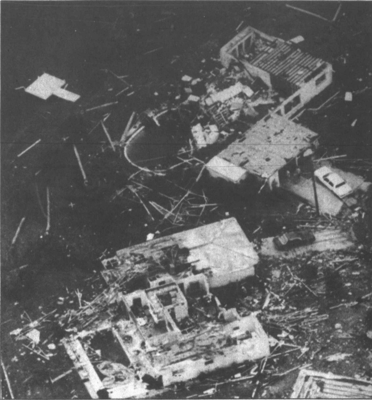
TORNADO DAMAGE —Several houses in Venice, Fla., are shown after a tornado passed through the area Sunday, injuring about 40 people and killing two. A Sarasota County Sheriff's Department spokesman said about 24 homes were destroyed and an additional 85 to 90 damaged. (AP Laserphoto)
