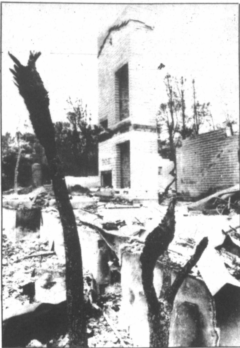
ALL THAT'S LEFT—A charred palm tree frames what's left of one of eleven homes destroyed by the massive Lexington reservoir fire near Los Gatos, Calif., Wednesday. Only the chimney remained at this home. Some 4,500 persons remain homeless because of the fire that has burned nearly 14,000 acres. (AP Laserphoto)
