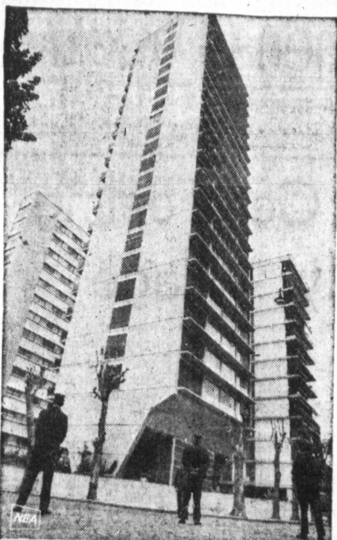
HIGH-RISE AND FALL in Buenos Aires. This apartment house complex in the Argentine capital's fashionable Belgrano district has been declared unsafe for occupancy. Police stand guard against return of evacuated tenants. In the last few months, at least two of Buenos Aires' modern skyscrapers have crumbled, killing 35 persons. Many other new buildings have been torn down after being condemned by the government. Nobody has yet determined or given an official explanation for the rash of collapsed buildings.
