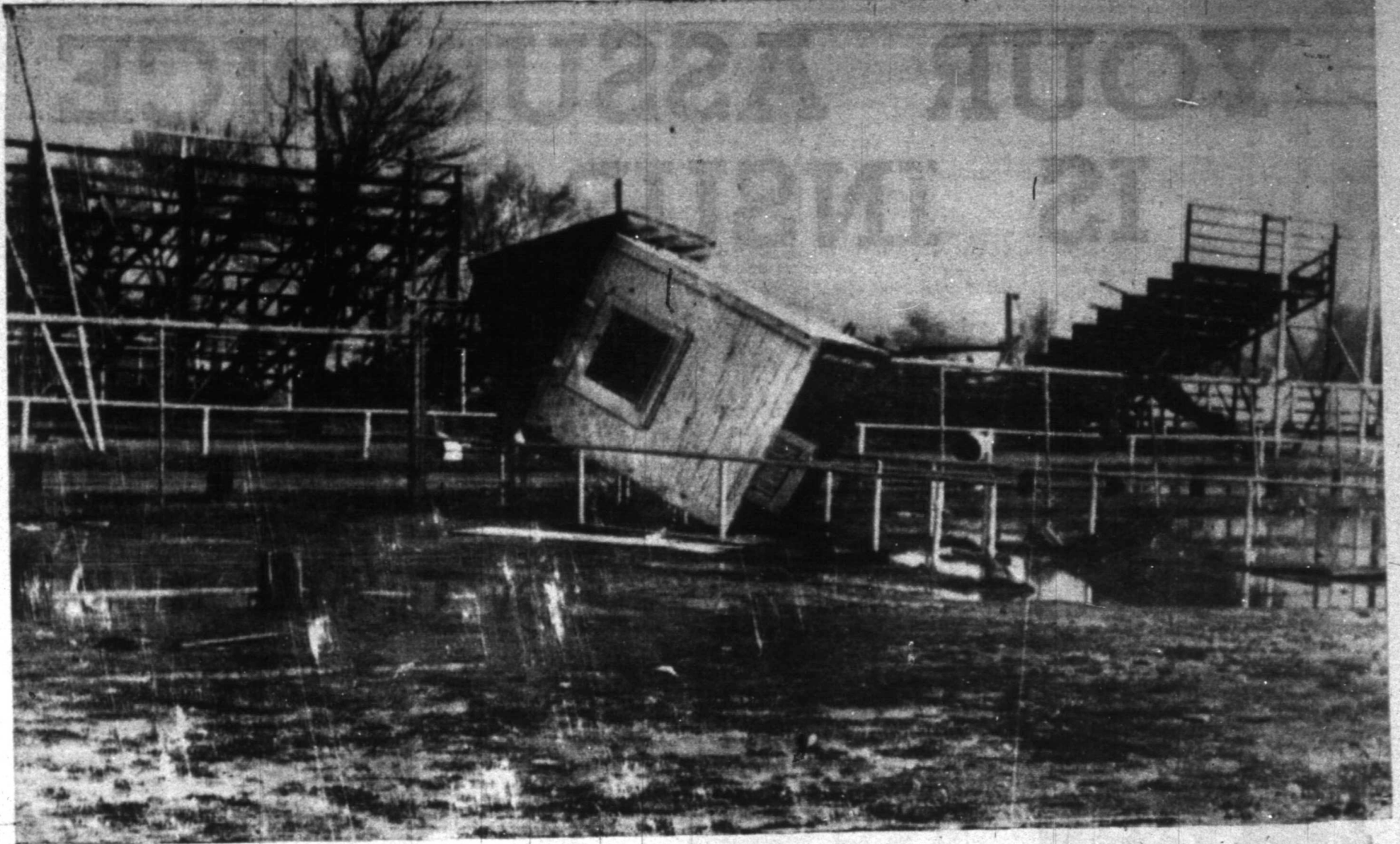
TICKET BOOTH at Top O' Texas Rodeo Arena entrance blown over and missing is one section of structure.
