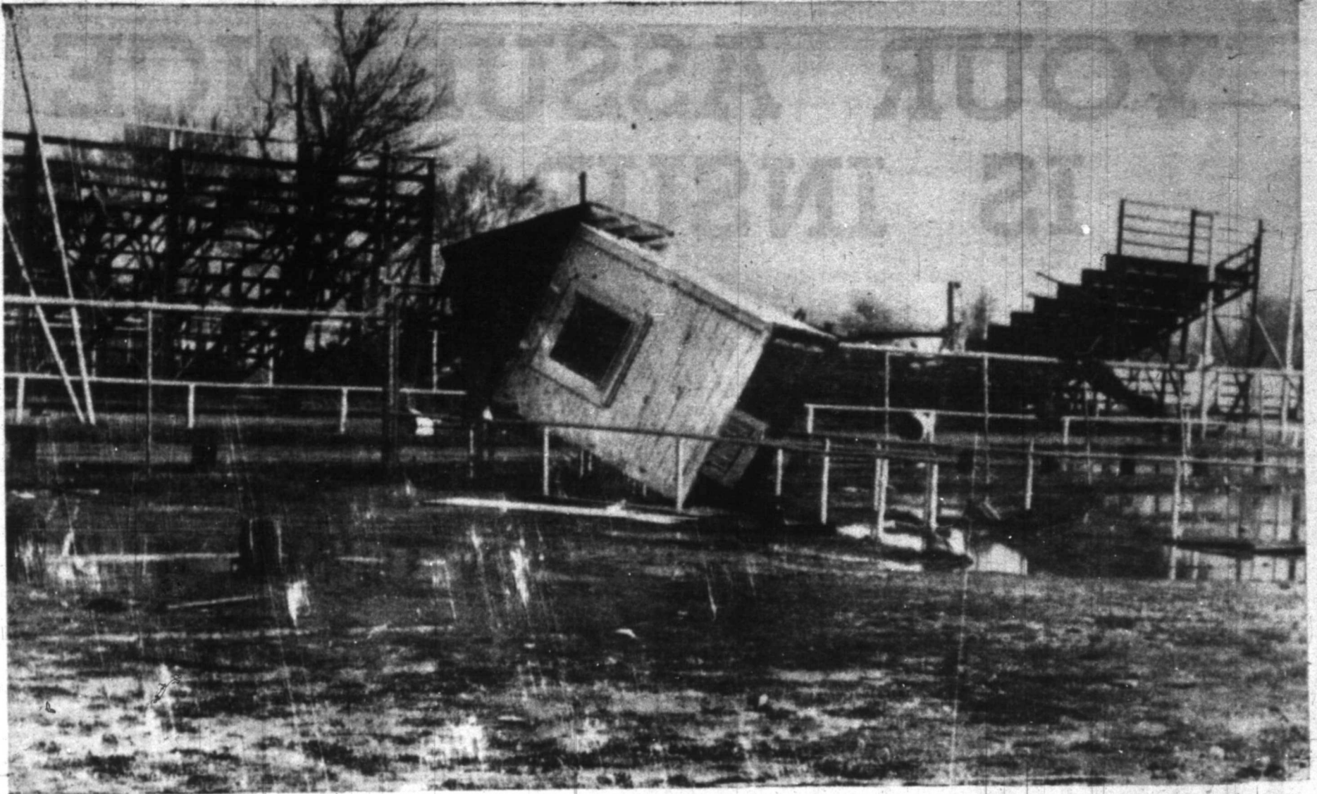
TICKET BOOTH at Top O'exas Rodeo Arena entrance blown over and missing is one section of damage.
