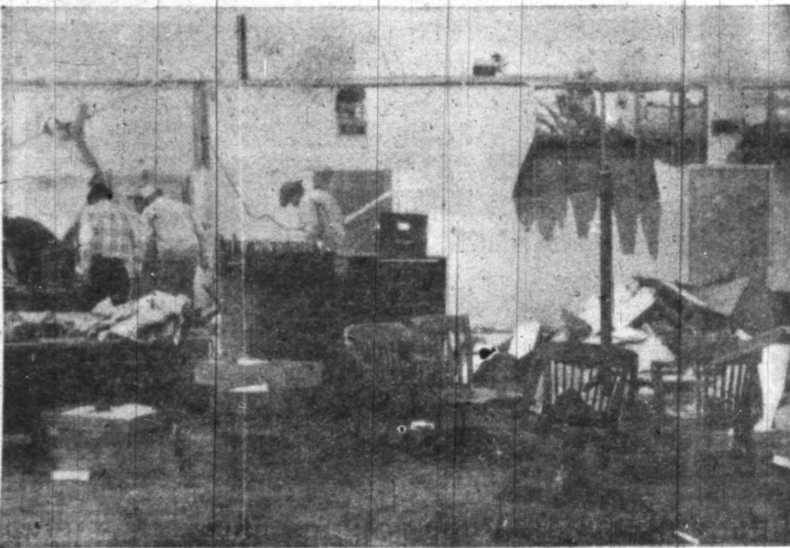
SCATTERED BY high winds, records and other contents litter the wall-less roofless county annex building east of town.
