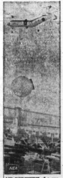
**AIR DELIVERY** of a one-piece fiberglass-reinforced plastic cooling tank on roof of a plant in Wilmington, Calif. It would have been costly to shut down the plant to move the equipment in, so a helicopter lowered the 1,800-pound vessel into position.
