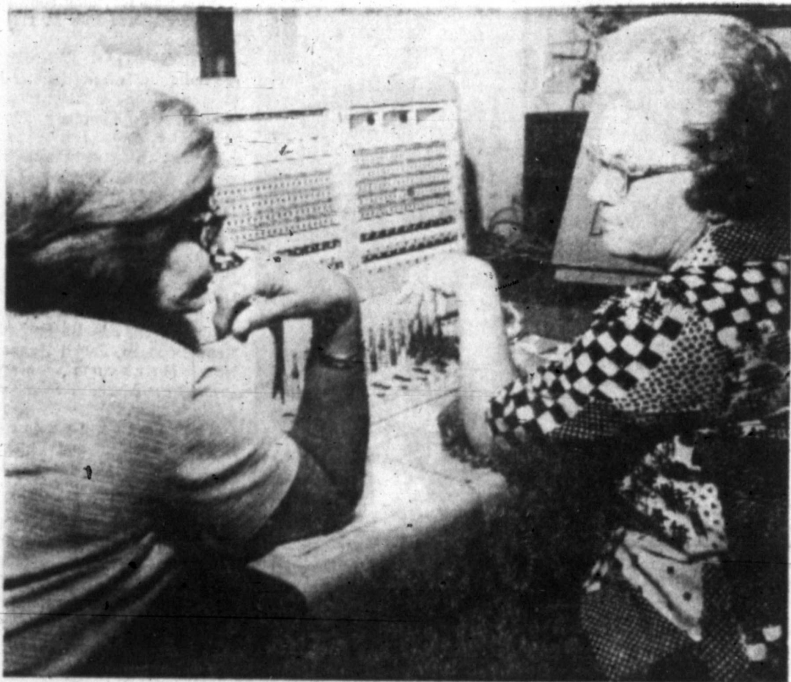
NEW SWITCHBOARD installed at Highland General Hospital keeps the communications organized. Mrs. Isabel Keith, Amarillo, left, a business service instructor for Southwestern Bell Telephone Co., instructs hospital operator, Mrs. Bun Hill, 1216 Garland, in the proper operation of the switchboard.
