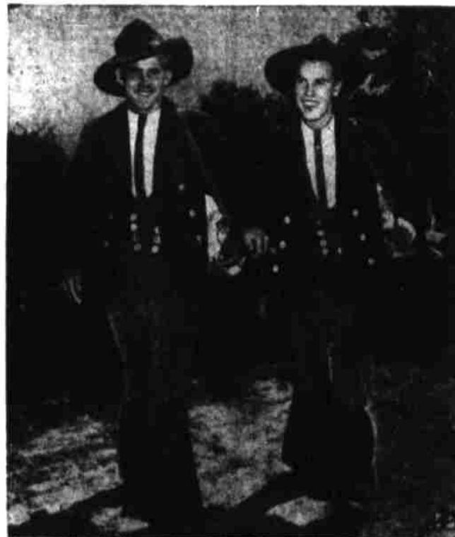
JOURNEYMEN-TO-BE —German mason apprentices, in 19th century costume, walk from Brunswick to Hamburg seeking work in revival of custom of changing jobs every six months.
