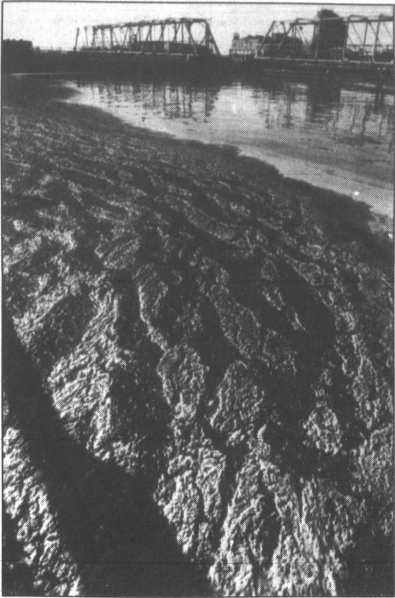
OVERWORKED SEWAGE PLANT —Waste matter collects in a sewage treatment plant in the Deer Island section of Boston. Every day, two overworked plants discharge 450 million gallons of wastewater and 100,000 pounds of partially treated human waste into the 47-square-mile harbor. When it rains, storm water laced with chemicals and raw
