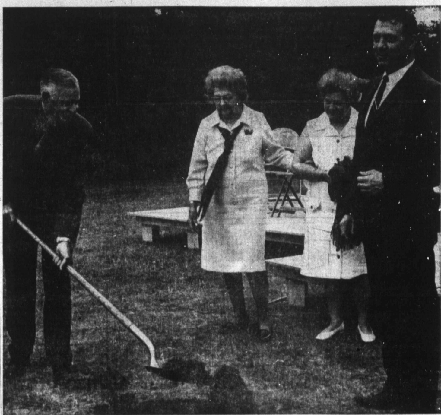
JOE GORDON, left, of Pampa, takes a turn at breaking ground in a ceremony at the National Cowboy Hall of Fame and Western Heritage Center in Oklahoma City Sunday, June 14, to begin construction of the Payne-Kirkpatrick Memorial, a new building at the Center to be constructed this year through the generosity of Mrs. Nona S. Payne, widow of the late David D. Payne, a pioneer West Texas rancher of the Pampa and Miami Texas area. Watching, from the left to right, are Mrs.
