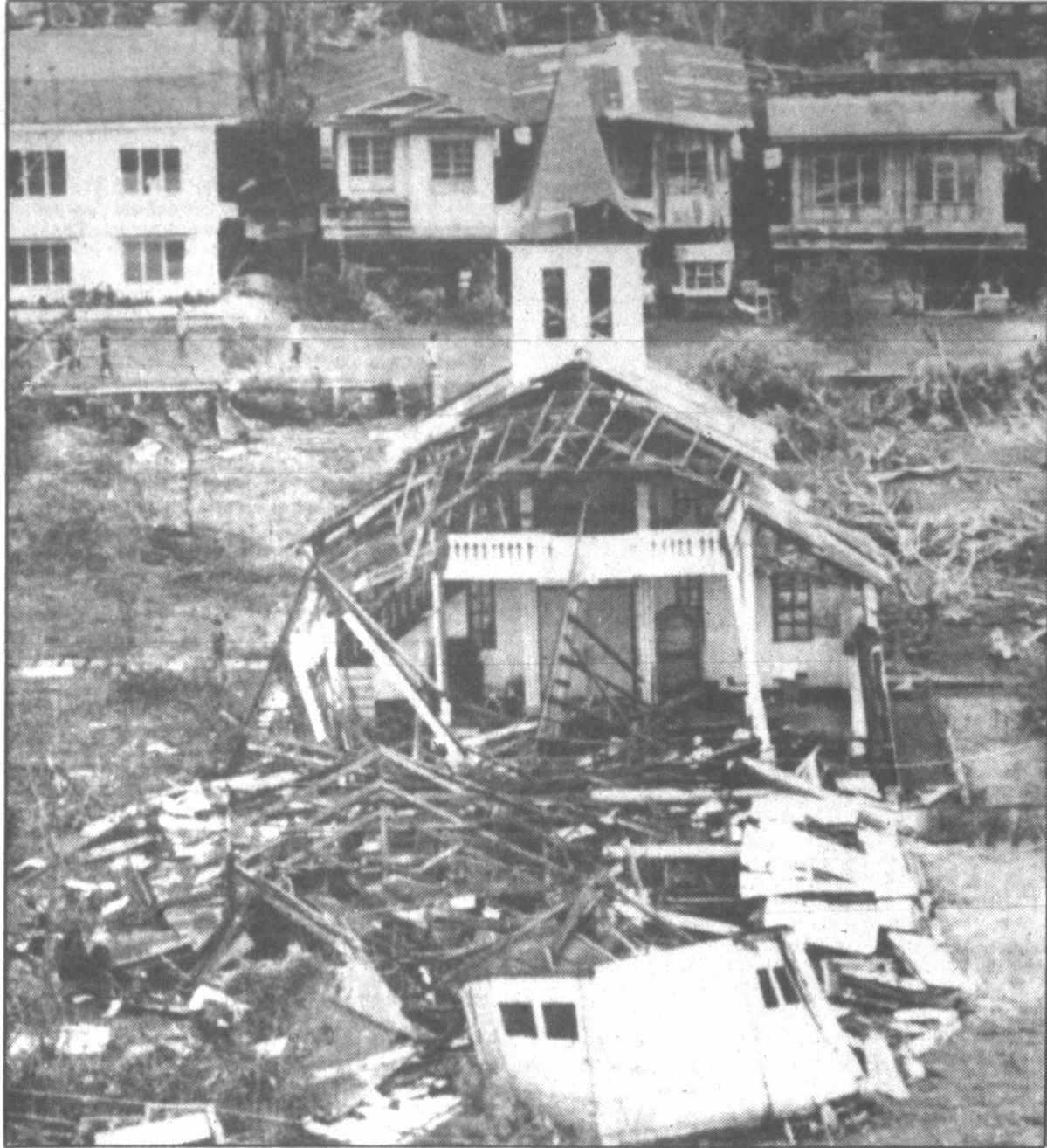
TYPHOON DAMAGE —Only the steeple shows that the collapsed building above is a church, one of the thousands of houses and buildings shattered by typhoon Ike's 115-mile-per-hour winds which battered the Philippines last weekend. The church is located in Surigao City, about 450 miles south of Manila. More than 1,000 people died and 200,000 others were homeless in the typhoon's wake. (AP Laserphoto)
