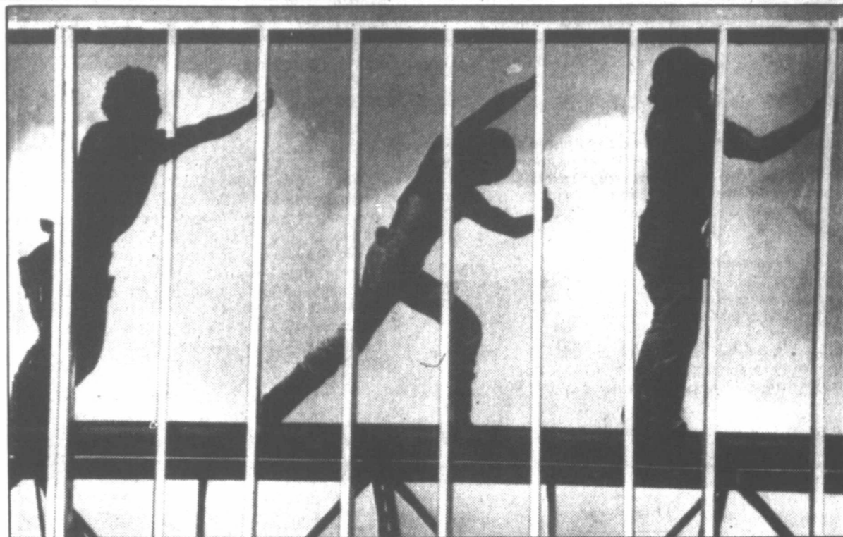
LINEAR CONSTRUCTION —Construction workers Mike Cortez, left, Jerry Gallegos and Scott Donner, right, straighten wall studs before bolting them together on a part of a new shopping center being built in Corpus Christi. (AP Laserphoto)
