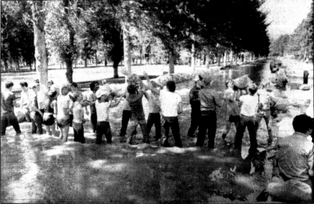
VOLUNTEERS RAISE DIKE —As temperatures in the mid-80s increased mountain runoff, volunteers turned out Sunday to bolster a sandbag channel through Salt Lake City's Liberty Park. The channel was created to divert a portion of the runoff into storm drains. (AP Laserphoto)
