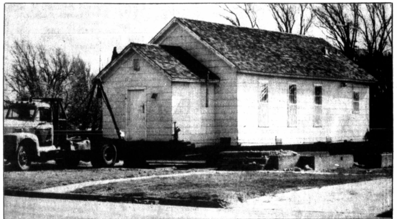
ON THE ROAD AGAIN - A building used by Zion Lutheran Church for Sunday School classes was moved Tuesday to a new location, one of many for the structure. The building was Gray County's first school building, erected in 1889. During its early history the school was shunted around several locations in the county while used as a school. In the 1940s it was moved into Pampa for use by the church. When the church embarked on a
