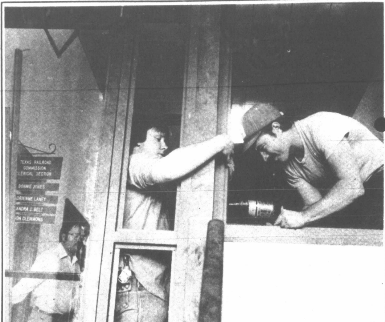
Renovation connects RRC offices
