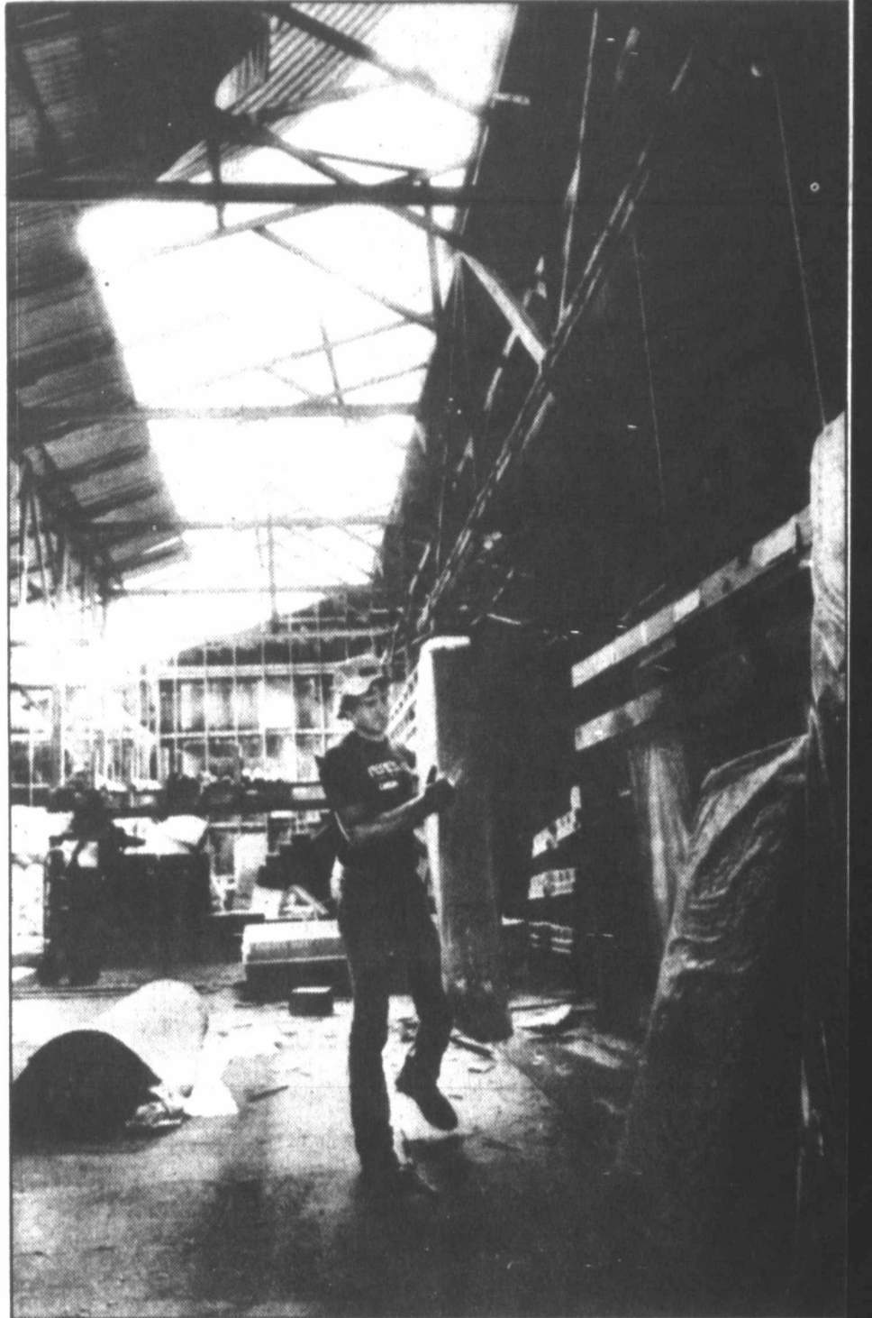
UNWANTED SKYLIGHT—Jimmy Coolbaugh moves some of the soaked merchandise to a more secure plane in the Higginbotham Brothers warehouse in Comanche Wednesday afternoon after a fierce wind and thunderstorm stripped the roof off the building Wednesday morning. Several commercial buildings in the Central Texas city lost their roofs and more when the storm struck. No injuries were reported. (AP Laserphoto)
