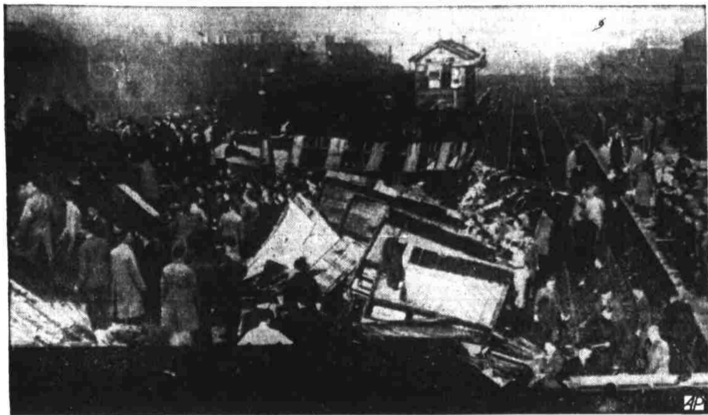
Wreckage Of Three Trains Outside London
