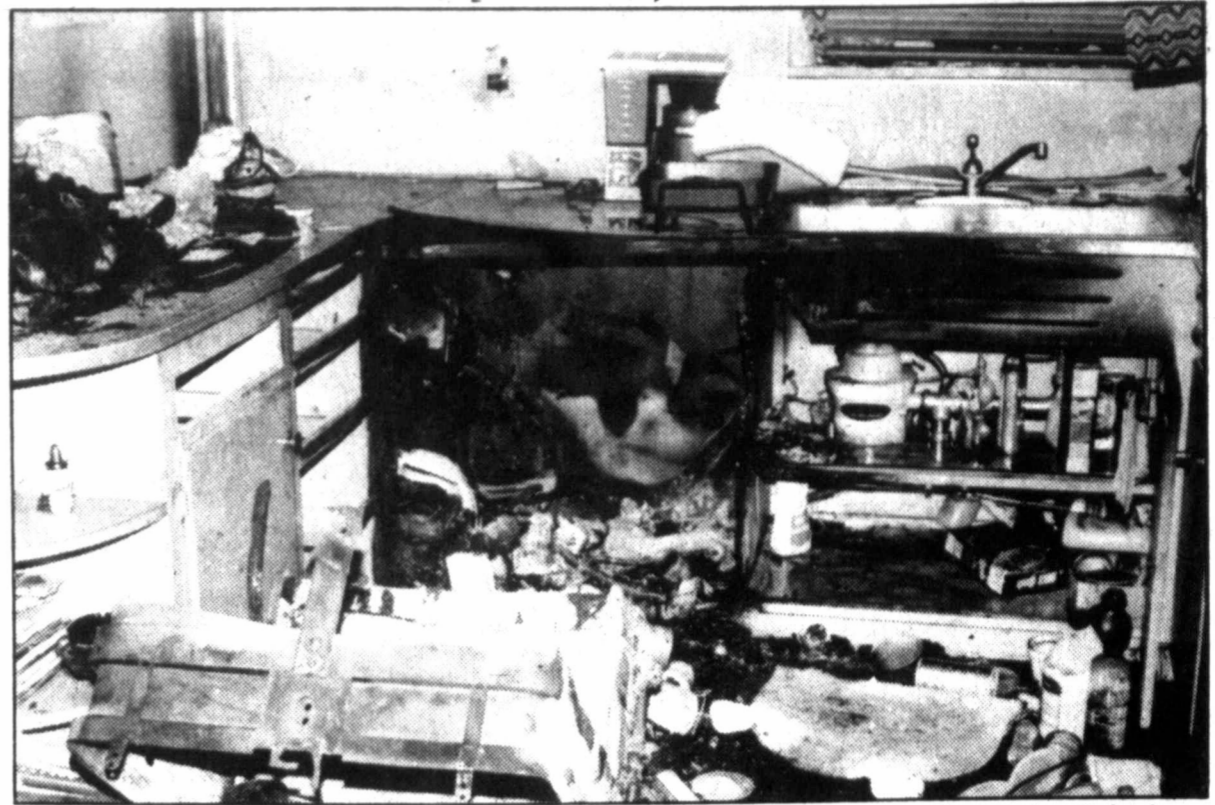
STRUCK BY LIGHTNING? — Pampa fire officials are uncertain about the cause of an afternoon fire that gutted the kitchen of the L.D. Hawkins residence, 1100 North Russell, although it was reportedly hit by lightning during a thunderstorm Tuesday afternoon. Nobody was home at the time and there were no injuries. (Photo by Ronnie Ledbetter)
