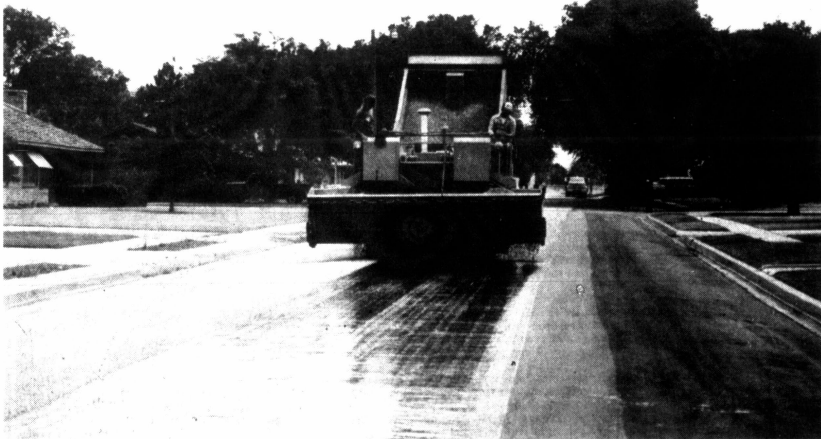
MOVING WESTWARD - Lewis Construction Co. crews lay down a layer of seal coating on Charles St. Tuesday afternoon before the rains came. The seal coating project moved onto Williston and Hamilton Sts. south of 23rd Ave. today. The crews will continue moving westward in the second week of the project. Forrest Cloyd, technician with the city
