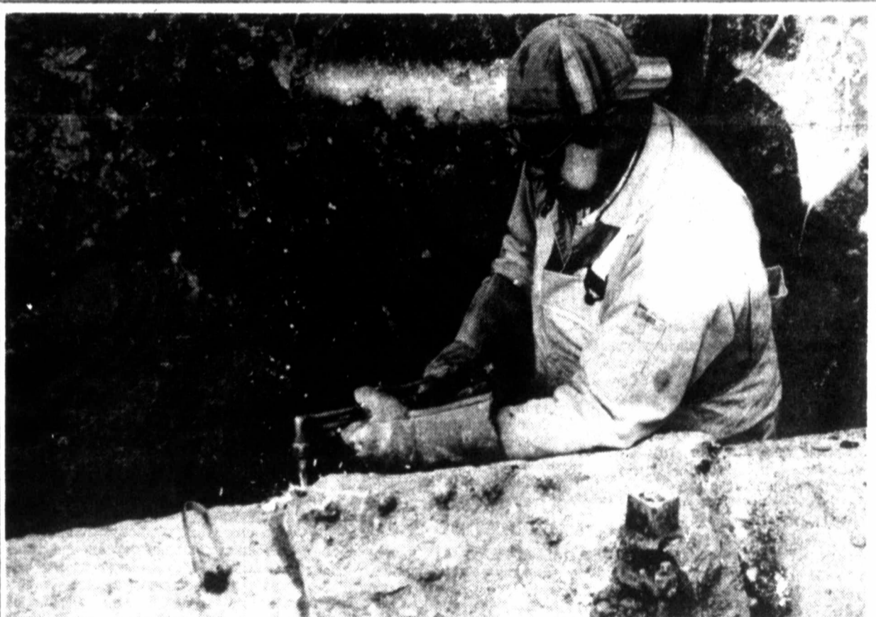
WATER LEAK REPAIRS - Phillip Alardin, employed with Gifford-Hill and Co. of Amarillo, cuts into a water distribution pipeline with a torch this morning to begin repairs on a leaking 16-inch tapping sleeve at the alley
