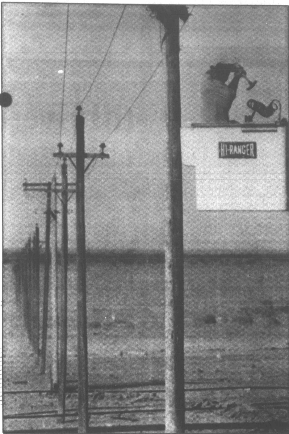
POLES TO POUND — Electrical worker Boyce Powell of Midland drives in the last spike to hold a crossbeam on a power pole that will take electricity to oilfield pumps near the far West Texas town of Texon, about 75 miles west of San Angelo. (AP Laserphoto)
