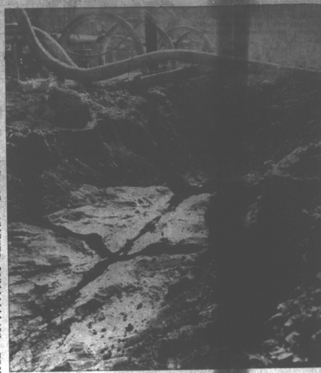
RIPPED-OUT — Tons of earth were blasted into the hole, some 20 feet wide at the top. Sections of the exploded pipe scattered around the area.
