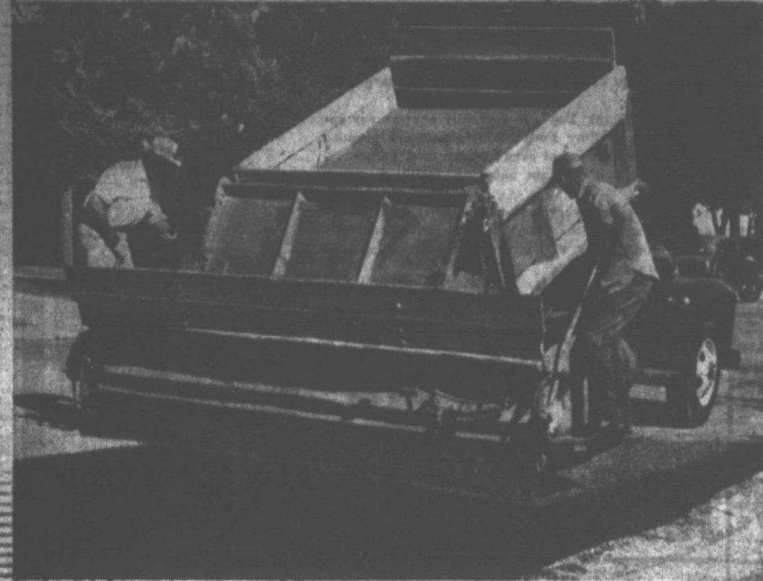
FIRST STREET — The 1100-block of North Somerville is the first street to be topped this season. Here a spreader box applies the topping. At the left is J. L. Riley, Canyon, job superintendent for Cooper and Woodruff, Amarillo, the outfit awarded the topping contract by the Pampa City Commission. To the right is J. E. McMillon, Post Oak, who operates the spreader box. Driving the vehicle (but unseen here) is Willie Mae Winters, Memphis. Other streets on which one or more blocks will be topped in the next few days are West Harvester, South Christy, Bradley Drive, Magnolia, North Warren, North Duncan, West 21st, East 21st, Dwight and Duncan. (News Photo)
