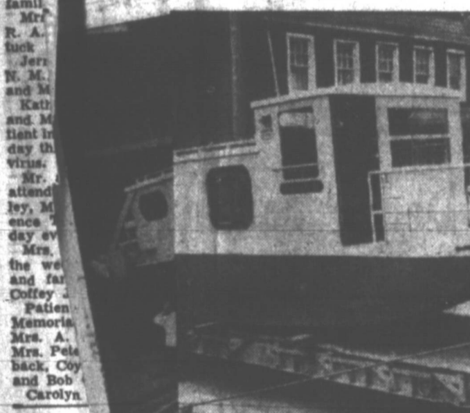
BOAT—After two years, Joe Burgard of York, Pa., finished his 32-foot houseboat. It's metal and resembles a house trailer without wheels. The floating "castle" is propelled by a chain-driven paddle wheel in the stern.
