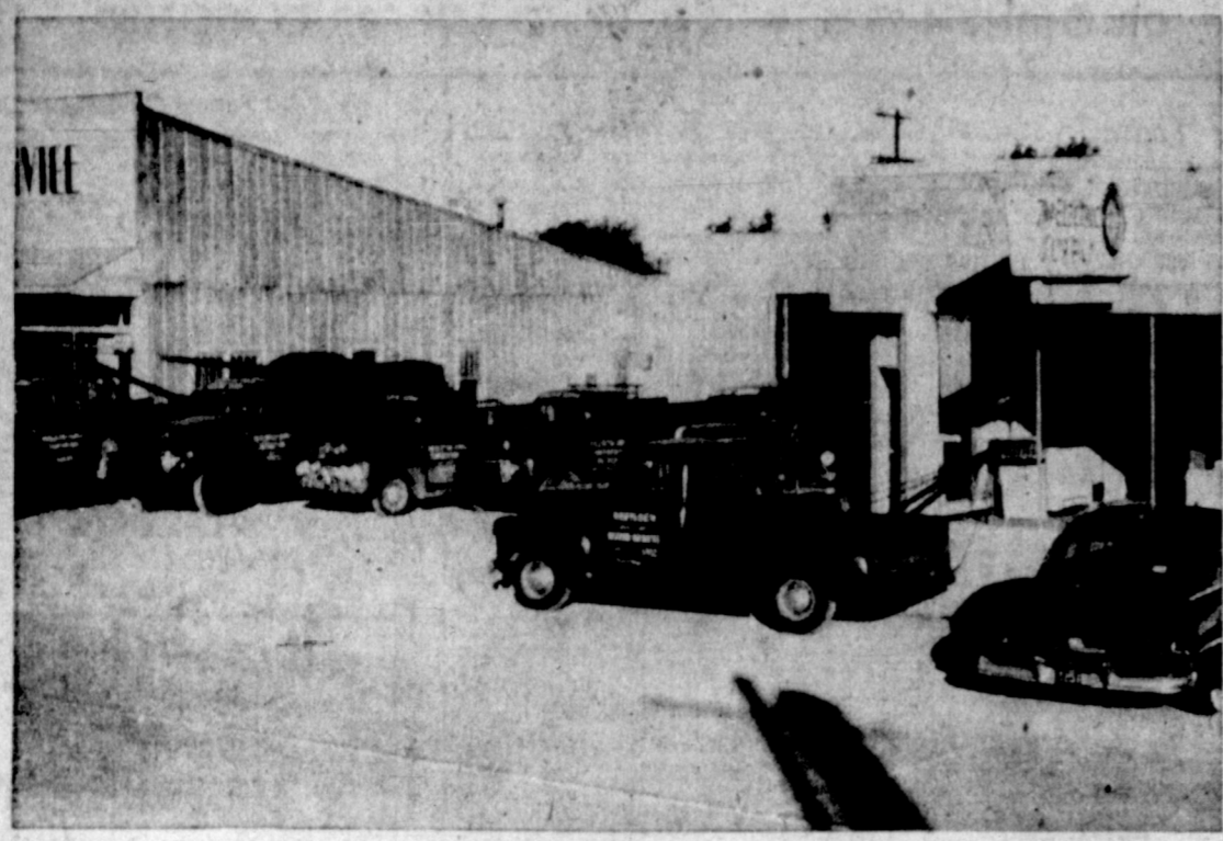
POISED TO SERVE YOU AND ELECTRICITY — Trucks of The Electric Supply and Dirksen Electric Motor Service, the motor repair firm associated with The Electric Supply, are lined up at 836 W. Foster just before they begin the day's work. All trucks are being equipped with 2-Way Radio to provide better, faster service.
