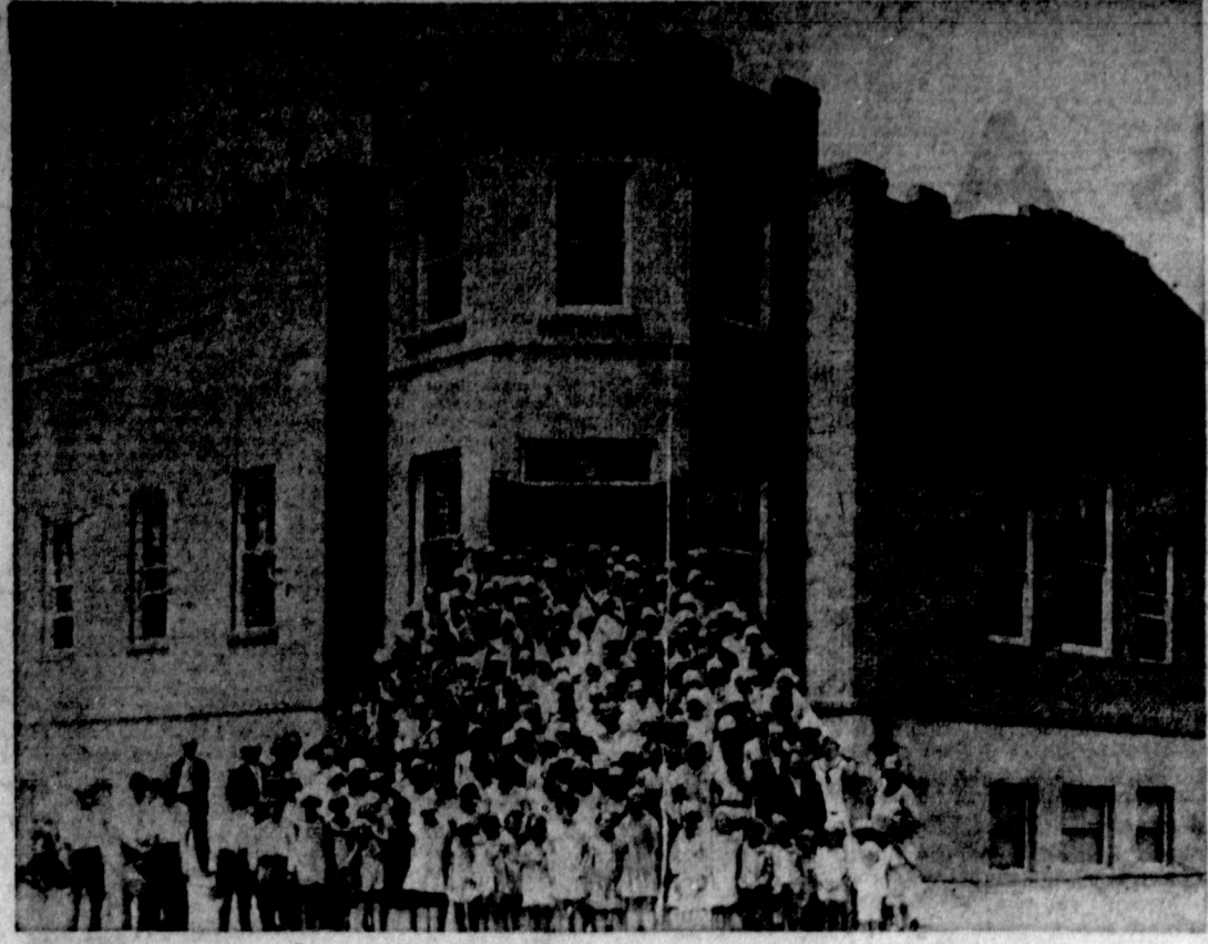
PRESENT McLean First Baptist Church consists of a sub-story, finished in 1923, a sanctuary, completed in 1929, and an addition and second story, added in the late 1940s.
