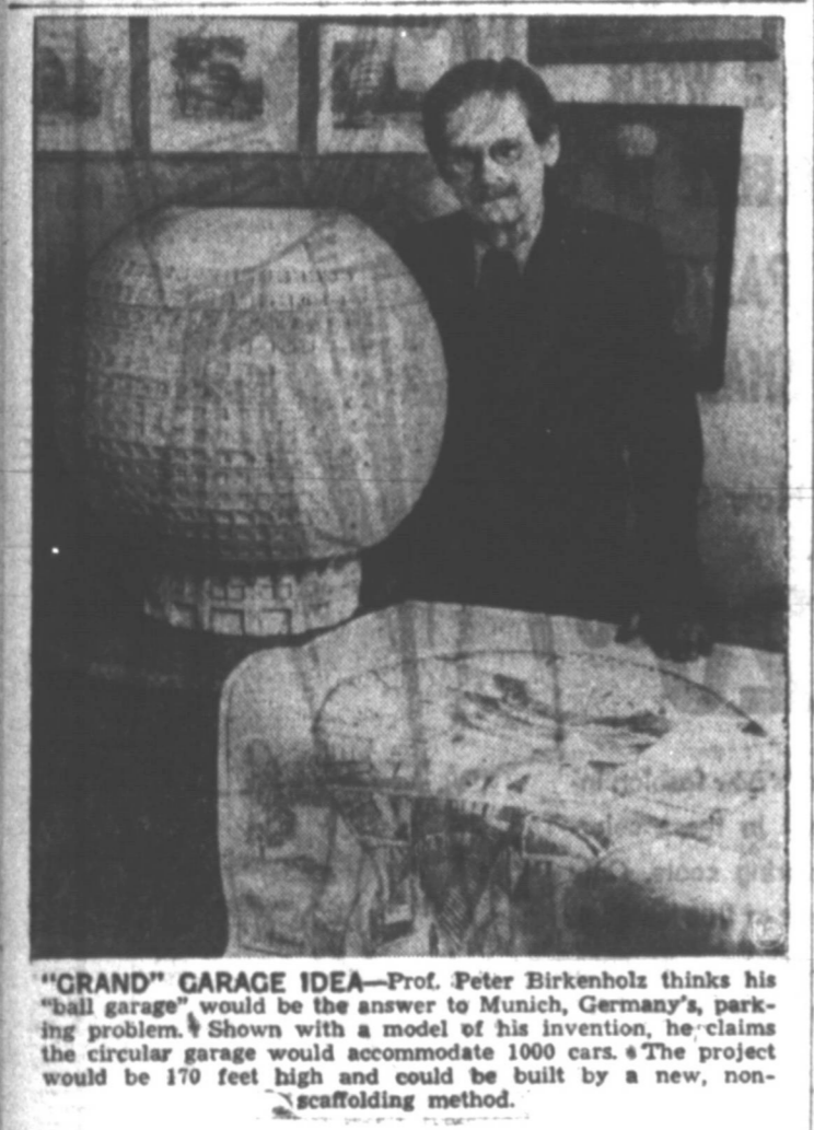
"GRAND" GARAGE IDEA—Prof. Peter Birkenholz thinks his "ball garage" would be the answer to Munich, Germany's, parking problem. Shown with a model of his invention, he claims the circular garage would accommodate 1000 cars. The project would be 170 feet high and could be built by a new, non-scaffolding method.
