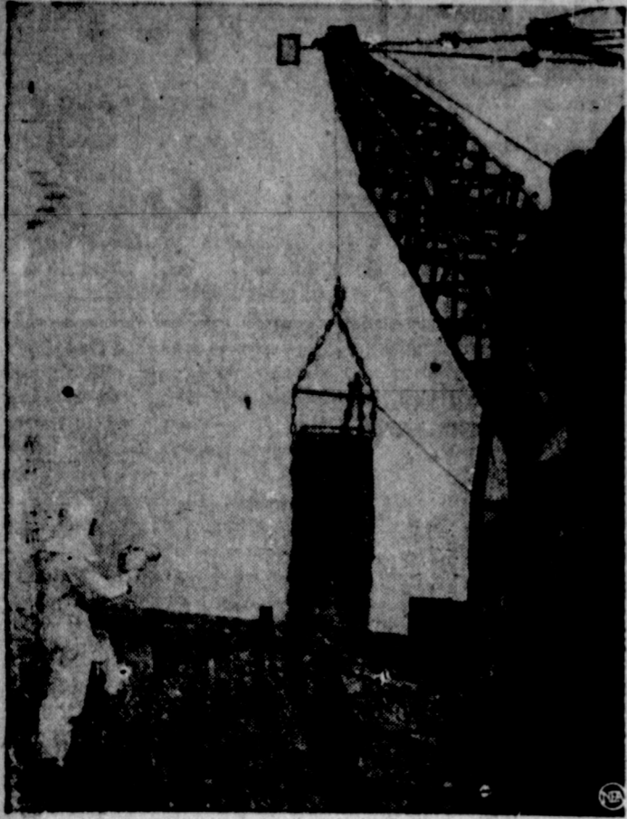
"BURIAL SUPERVISOR" in hooded suit keeps track of radiation as dragline covers atomic casket with dirt. Mirror on boom gives operator view of grave beyond earth and concrete shield.
