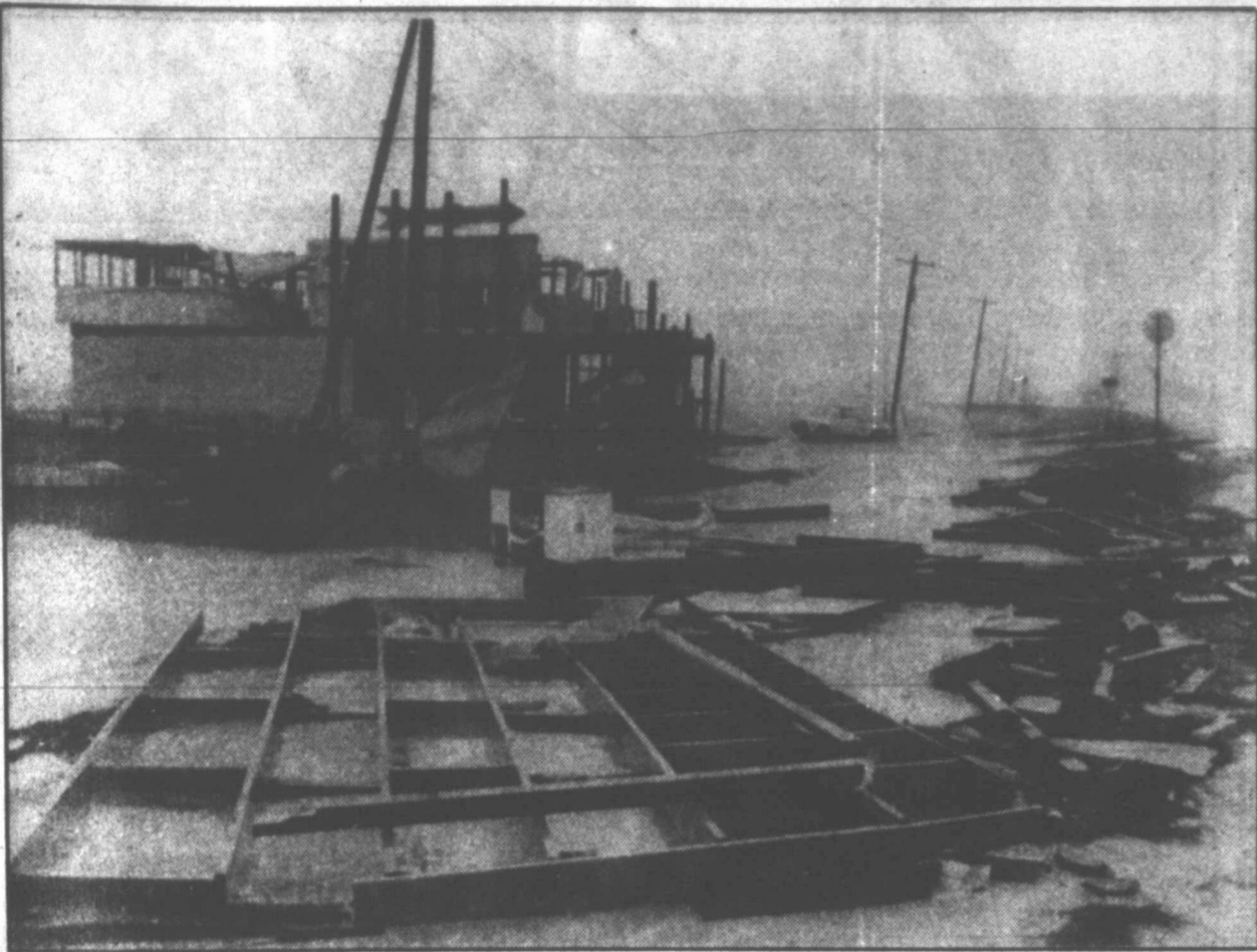
A store at Surfside Beach near Freeport was torn apart by Hurricane Alicia Thursday morning as the storm moved inland. Alicia came ashore with 115 mile an hour winds. (AP Laserphoto)
